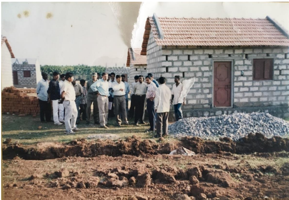
MC Halli site inspection by Yatish Kumar with the DC and other officers during Bhadra relocation. Photo credit : D V Girish
