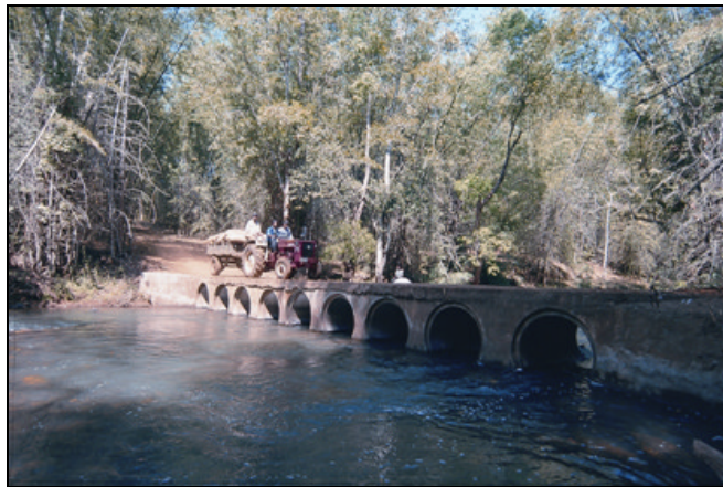
Bridge constructed by project proponents over a perennial stream inside BWLS to ease transportation for the local people
